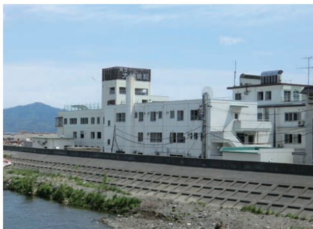
■ Photograph 3: Old Iwate Prefectural Otsuchi Hospital
