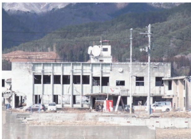
■ Photograph 2: Old Otsuchi Town Office
